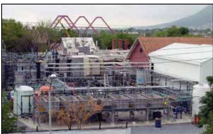
Peñoles, Mexico demonstration bioleaching plant built by BacTech
